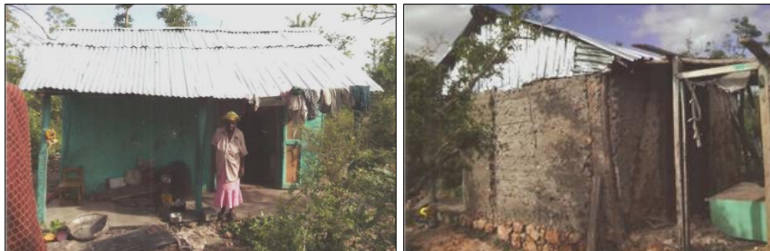
Mme. Madeleine Etienne's new home (no before pictures because house was leveled)
